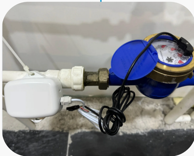
Pulse output watermeter + plug&play pulse counter (no need electricity. works with battery)
